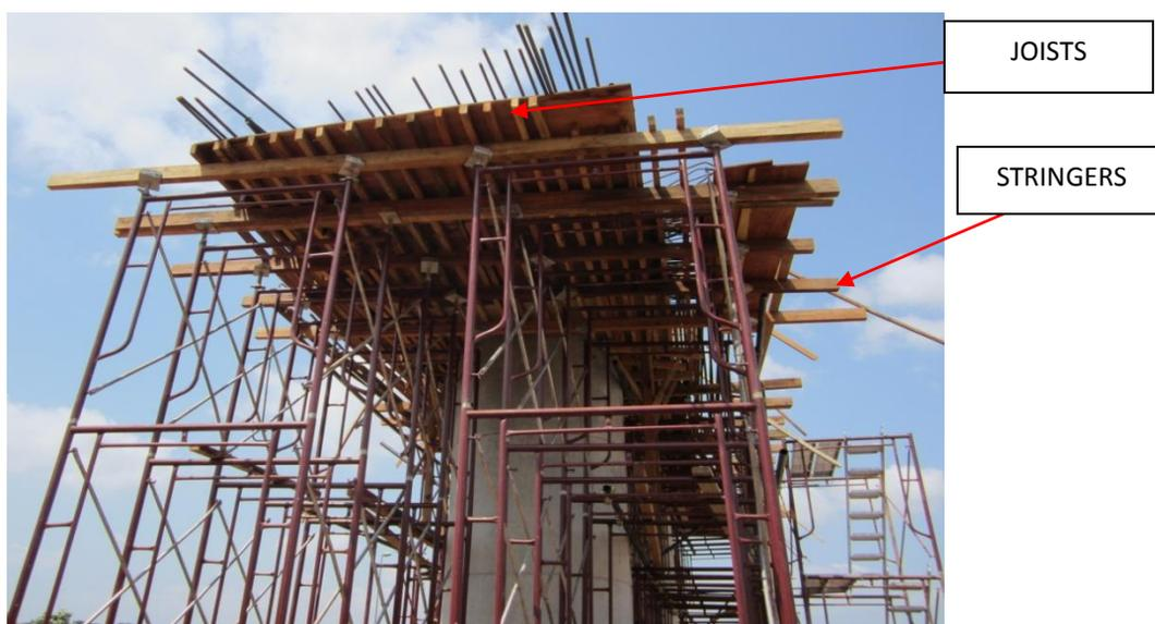
Figure 1: Timber formwork for concrete bridge crossbeam construction.
