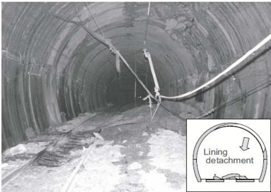
Figure 1: Damage to the Wanatsu tunnel
