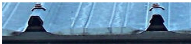
**Figure 2.5:** Klip-Lok Roof Sheeting.
