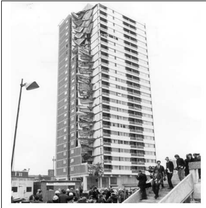
Figure 2.2 – Ronan Point Building after 16 May 1968 collapse [2]
