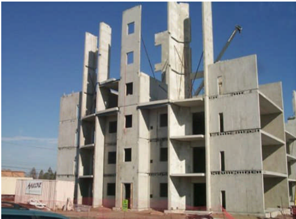
Figure 2.1 – Wall – Slab Frame Precast System
