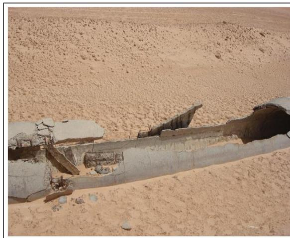
Figure 1: Reinforcement corrosion and the bursting of the cover concrete sanitation pipe N'Goussa - Ouargla.
